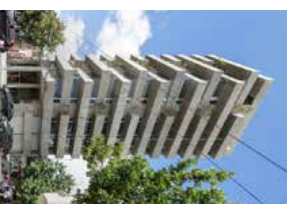
Fig. 6.2.26 Building Pleyredon 1101 Source: Estudio Pablo Gagliardo, 2017
